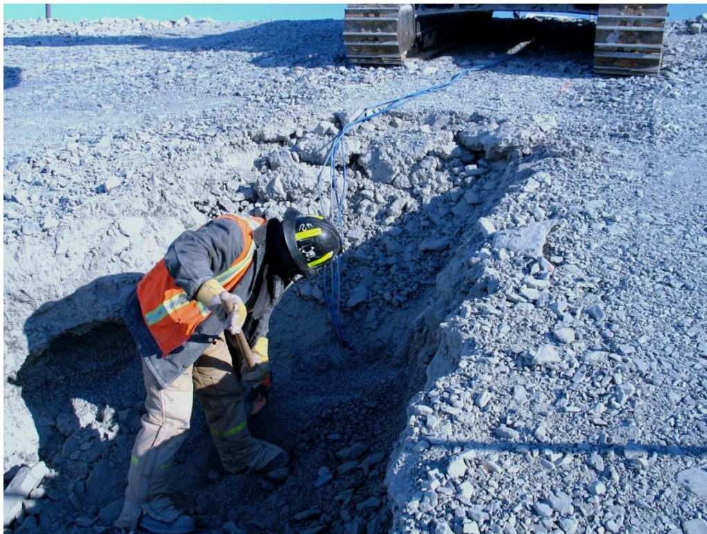
Photo 9: Sta 0+85 End of severed cable
