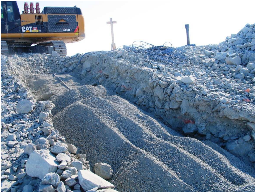
Photo 6: St 0+85 Near the top. Wide trench resultant from using a large bucket.
