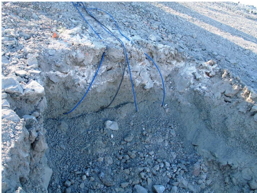
Photo 2: Cable layout at Sta 0+85 necessitated hand excavation under each. Cable on left was the severed cable
